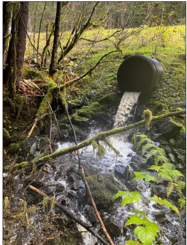
Figure 3.—Perched culvert outlet at waypoint 1030.
